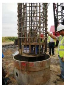
Installation of pile cage with O-cell assembly
